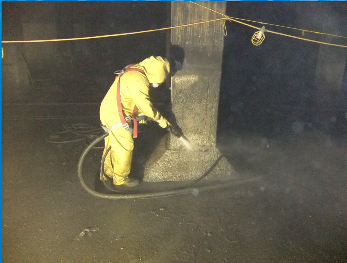
Sand blasting to prepare concrete
