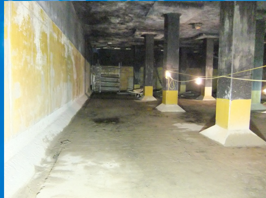
Tank condition before rehabilitation
